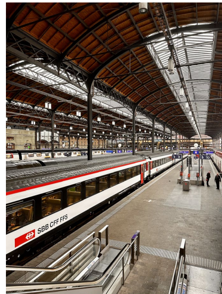
Figure 2 - Basel SBB Train Station
